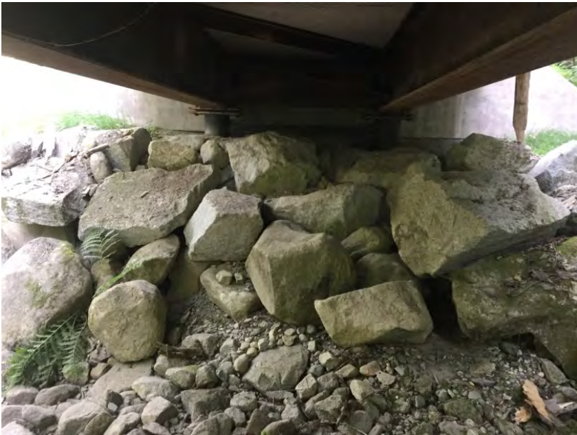
Right Bank Abutment when facing downstream
