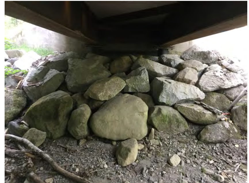
Left Bank Abutment when facing downstream
